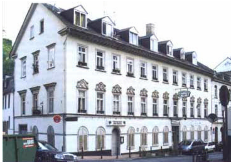
Ill. 3: The Pariser Hof Bathhouse, 1999
